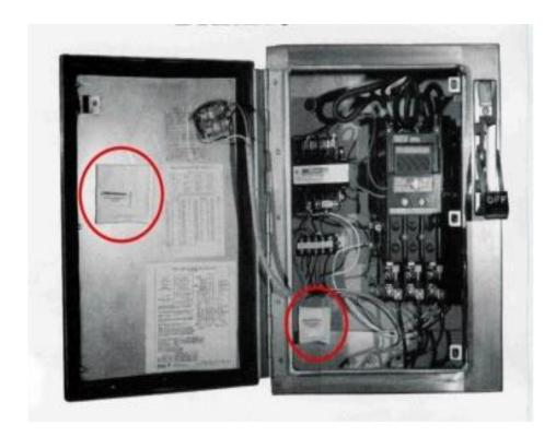
H2O Moisture Control Packets are desiccating bags developed to combat moisture caused damage that occurs in enclosed areas. The unique design of the packets captures water on a microscopic level, preventing corrosion. Once activated the packet will become Swollen indicating replacement is required.
